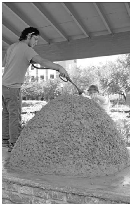
A student waters down the cob oven in its early phase.
